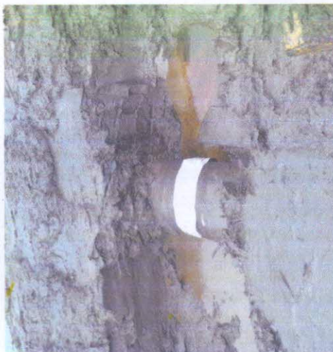
Fig C: picture taken after wrapped.
