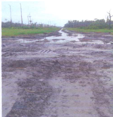
Fig D: picture taken after backfilled.
